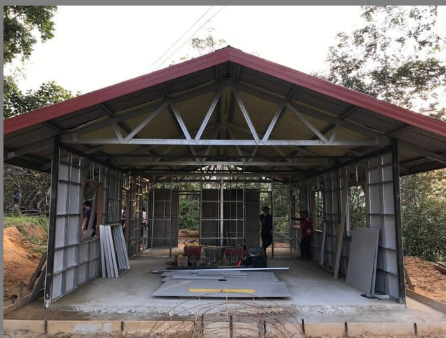
Figure 32: Wall studs overview.
