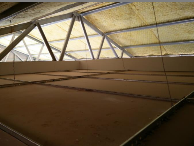
Figure 38: Ceilings suspended from the battens
