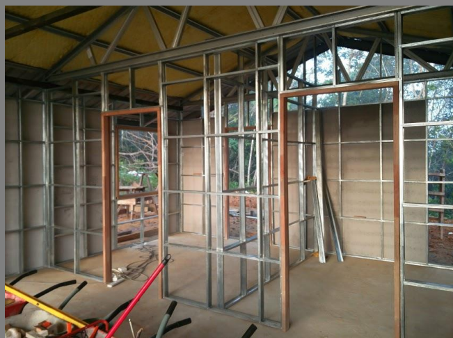
Figure 33: Internal wall studs
