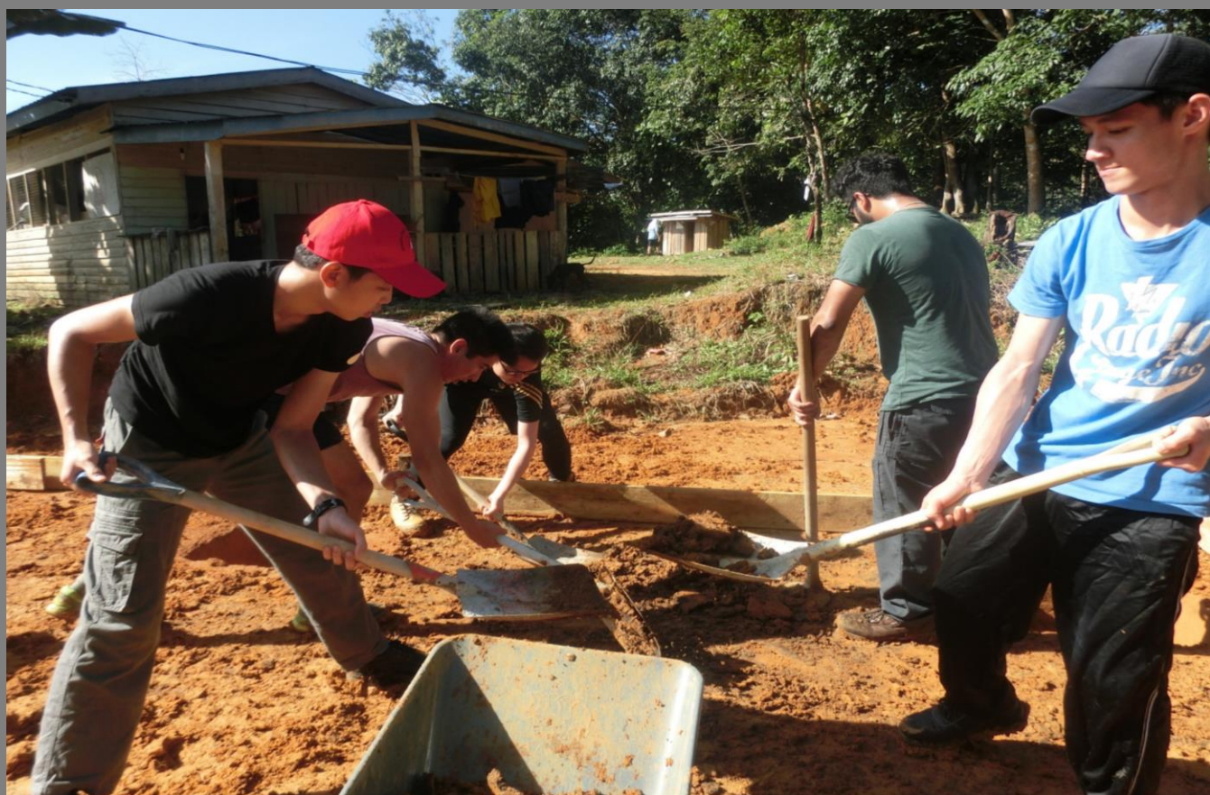
Figure 22: Site levelling
