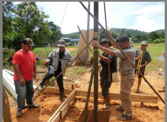
Figure 21: Column propping
