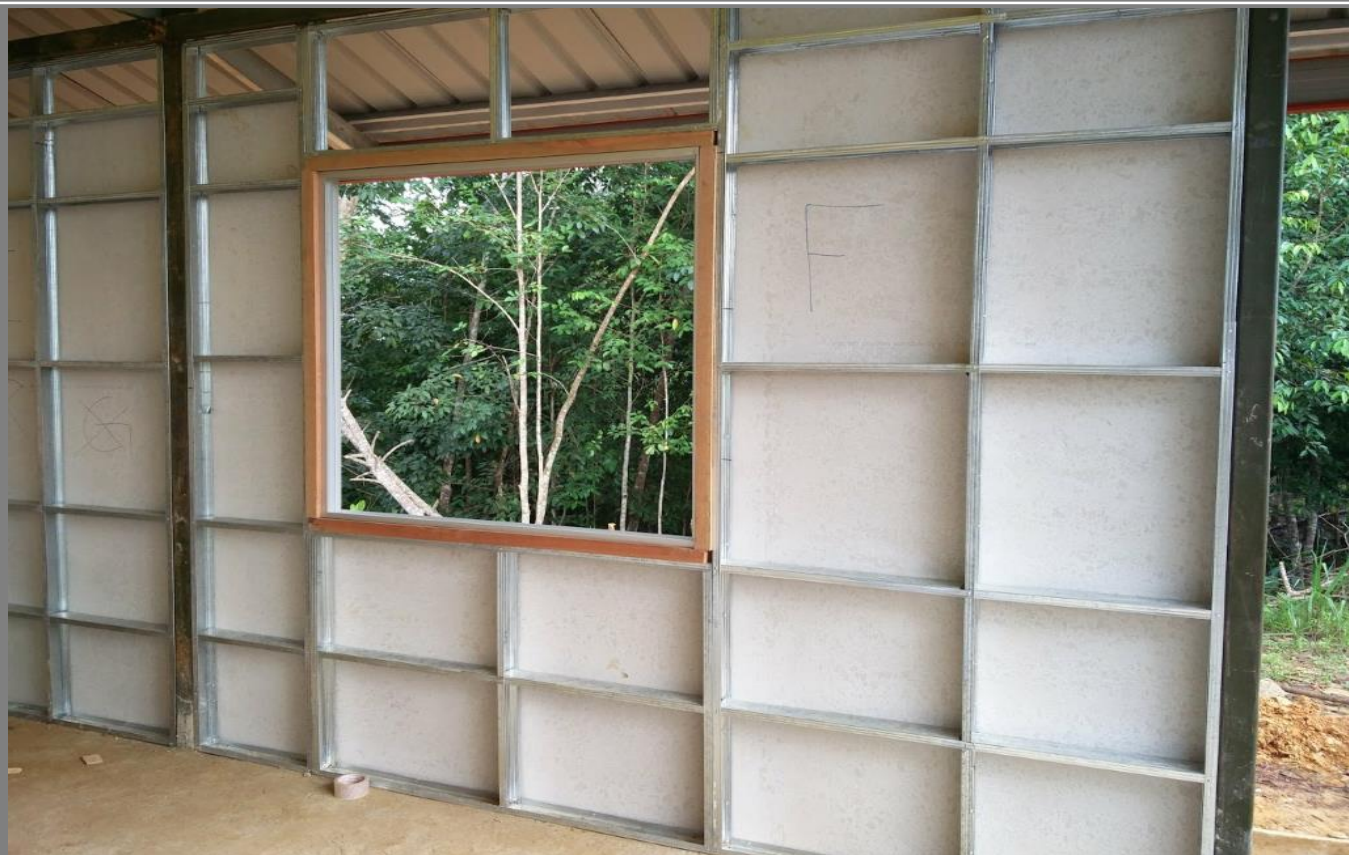
Figure 31: Wall panels attached onto the wall studs.
