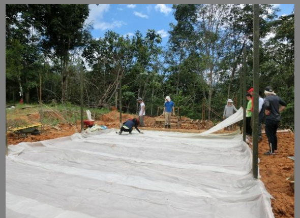
Figure 27: Concrete slab water proofing.
