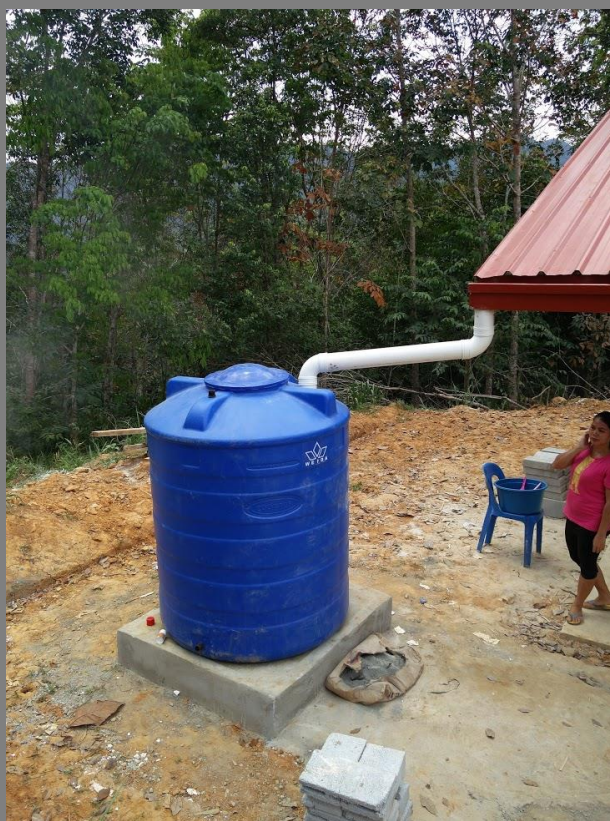
Figure 41: Rainwater Harvesting System
