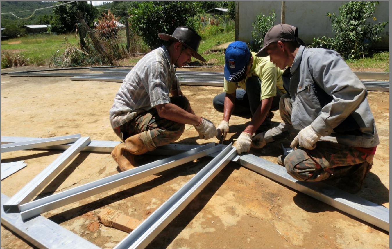
Figure 25: Truss assembly.
