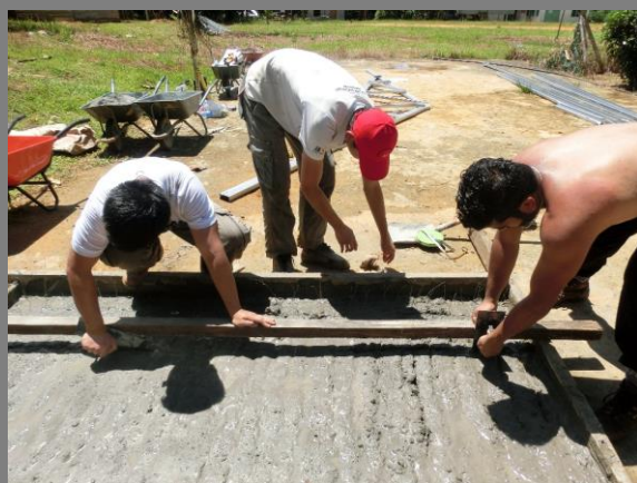
Figure 23: Spacer making
