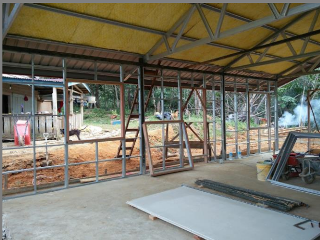
Figure 29: Wall studs.
