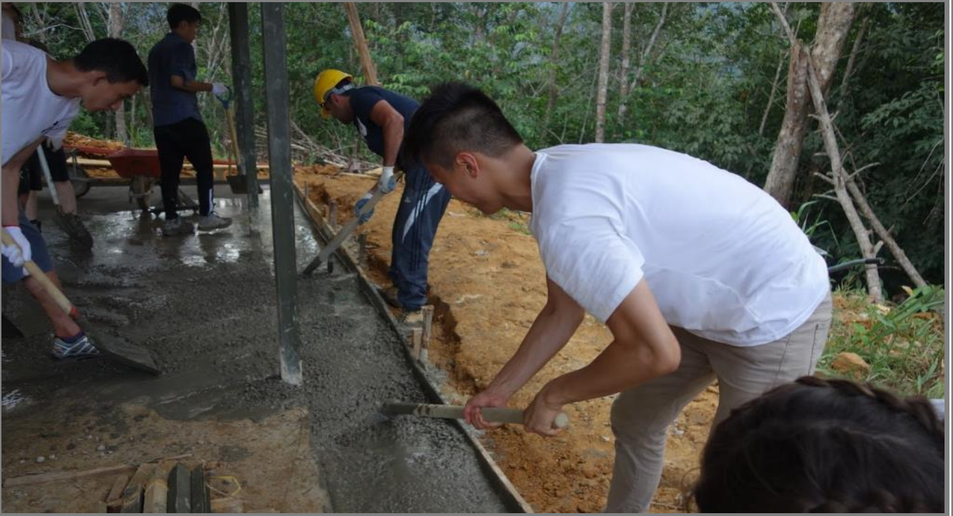
Figure 28: Casting of the outerslab.
