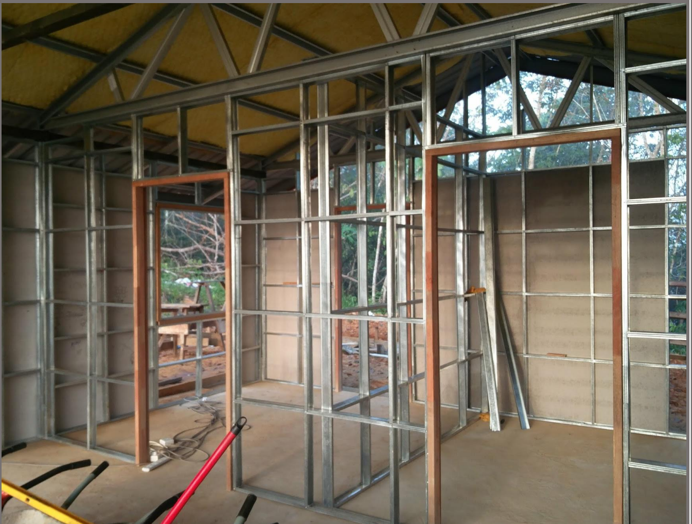
Figure 13: Internal wall frames of the kindergarten.
