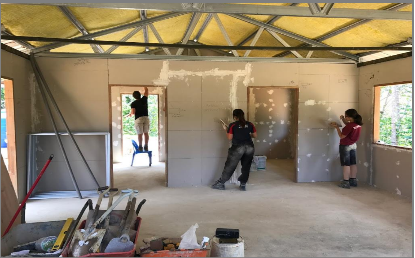
Figure 37: Plastering the wall panels.
