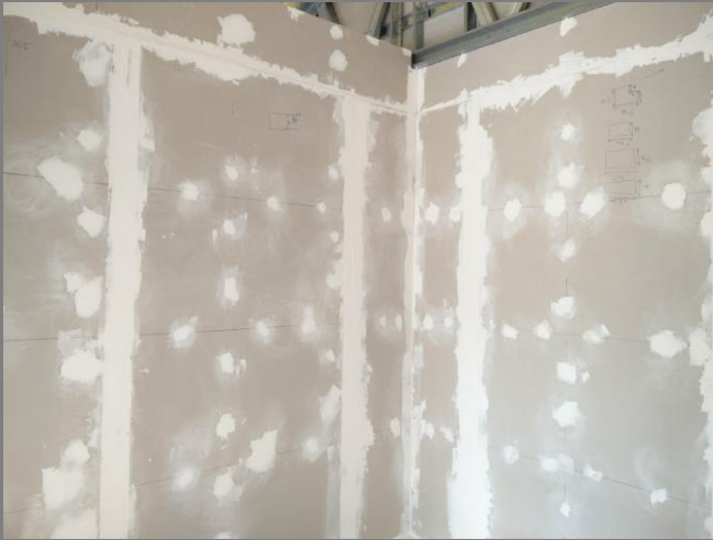
Figure 37: Plastering the wall panels.
