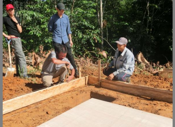
Figure 20 Setting out.
