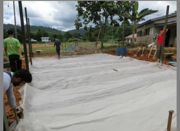
Figure 26: Polyethylene sheets positioning.
